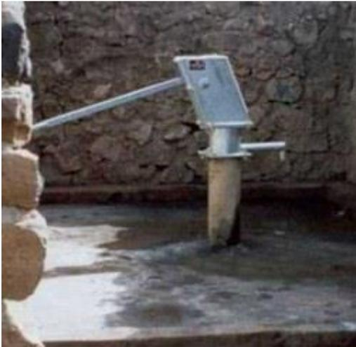
The India Mark III Pump is a robust conventional lever action handpump for shallow to medium deep wells. It is designed for heavy-duty use, serving communities of 300 persons. The maximum recommended lift is 30 m. Besides the “Standard 63.5 mm” configuration, there exists a version with Ø50 mm cylinder size for lifts up to 50 m.
